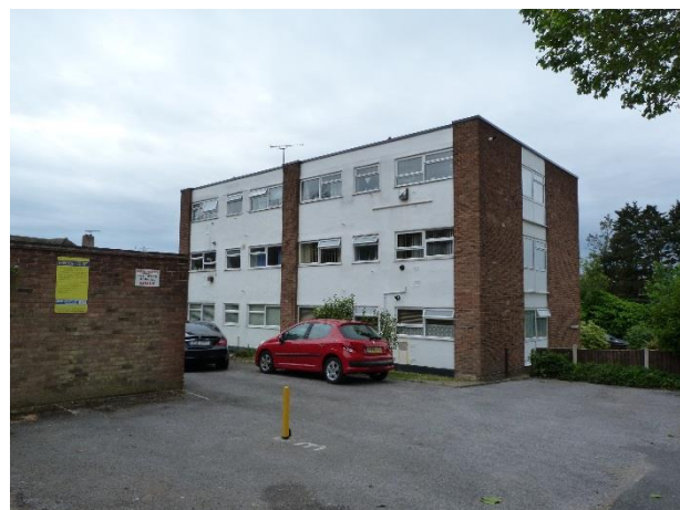
Poor quality modern infill at the southern end of Preston Road
