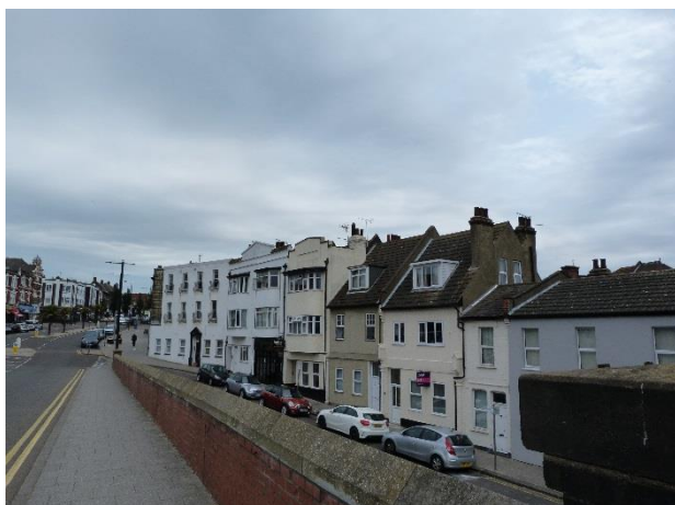
Buildings rendered and painted, with uPVC window replacements, at the southern end of Hamlet Court Road
