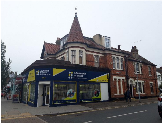
Examples of inappropriate shop fronts
