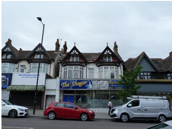
Example of poor shop fronts
