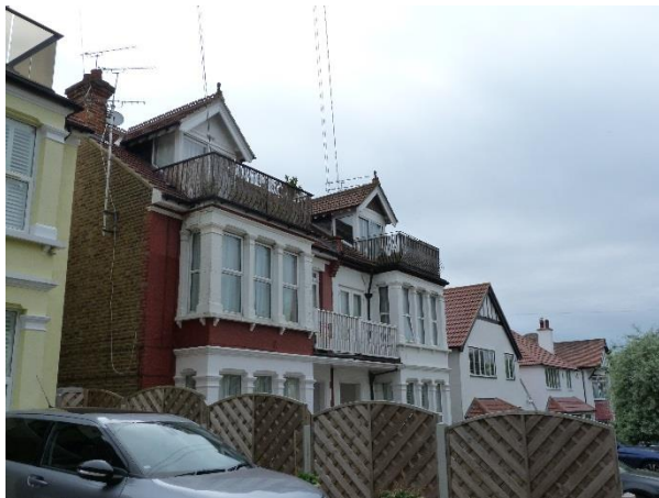
Variety of designs and inappropriate alterations on Cossington Road
